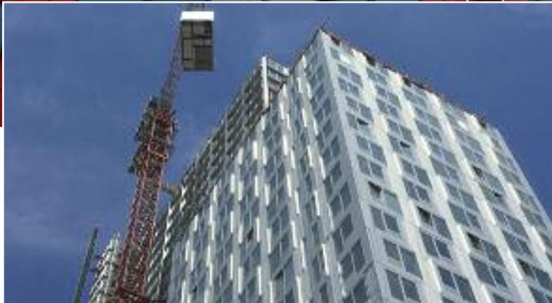
**Modular building offers an efficient, quality driven alternative to traditional construction.** More and more companies are using this design and construction process because it offers greater time and cost predictability with the use of repetitive components that make it easy to calculate project timeline and cost. Eighty percent of construction occurs off-site resulting in fewer deliveries and reduced neighborhood impact.
